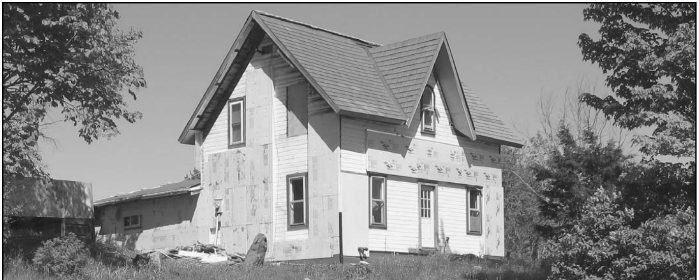
The George Slack Home, 101 Black Rapids Road, as it looks today. (See Recollections & Reflections - Pg. #5) Photo by Bill Boulton
