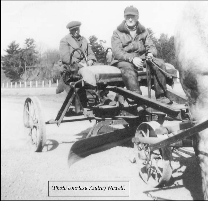
Phil Hunt and Kenneth Hill grading road bed with horse drawn grader
