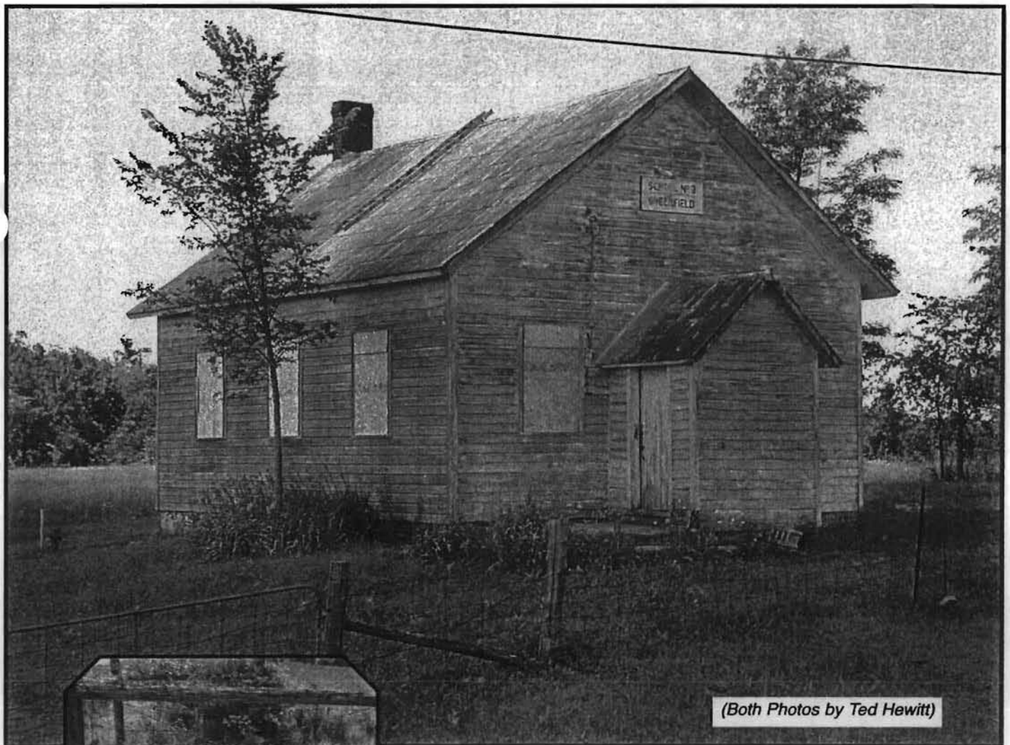
Restoration of Greenfield School as of late June, 2000. The original well is shown in the inset photo- see cover photo issue #12
