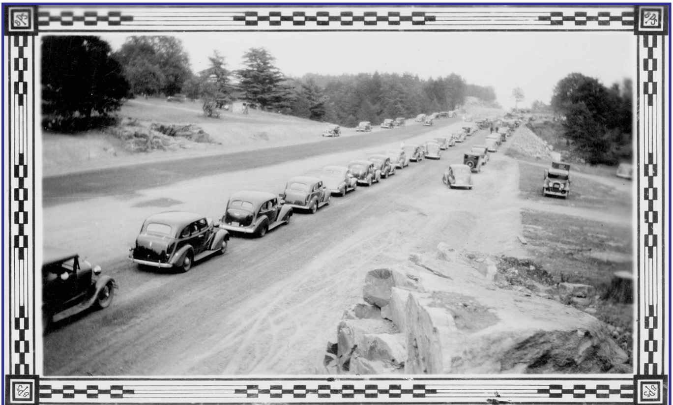
Line of Cars at Bridge Opening - Photo Courtesy Glendine Landon
