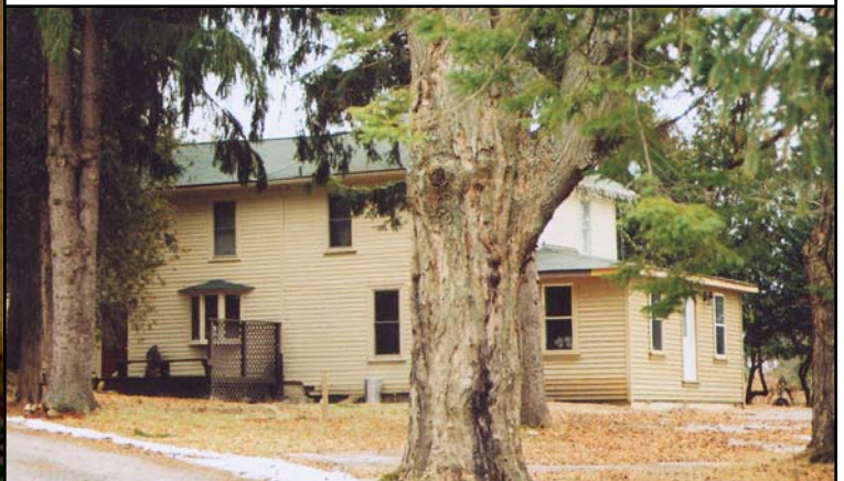
72 Flags Creek Crescent. Location of the shooting as it looks to-day
